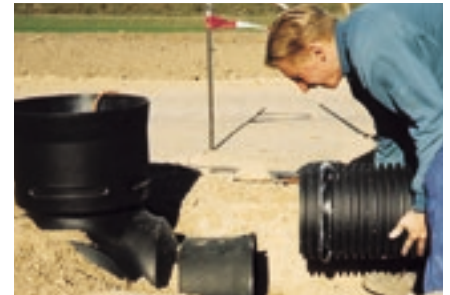
Its low weight facilitates installation. Matching accessories meet all the demands that are placed on easy-to-install drainage technology.
