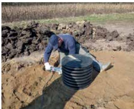
If necessary, extension pipes can be cut to length in the middle of corrugation troughs using a fine-toothed saw or a pipe cutter.
