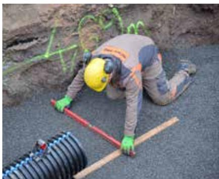
Create the excavation pit according to the planning specifications. The provisions of DIN 18300 "Earthworks" (*Erdarbeiten*) and DIN 4124 "Excavations and trenches" (*Baugruben und Gräben*) apply. When installing the shaft, comply with DIN EN 1610 "Construction and testing of drains and sewers" (*Verlegung von Abwasserleitungen*). Create and compact a planar shaft bearing with 10 cm to 15 cm of stoneless, compactable material.
